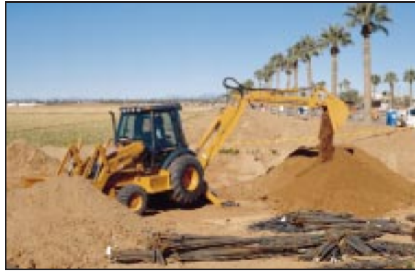
Vehicle monitoring includes not only passenger cars, but locomotives, airplanes, helicopters, tractors, buses, heavy trucks, drilling rigs, race cars, and motorcycles. (Photo courtesy Case Corporation.)
